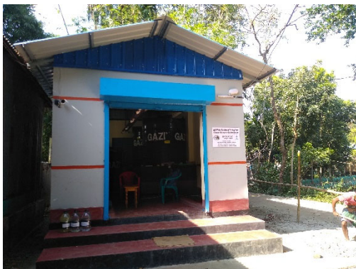
External appearance of plant constructed
